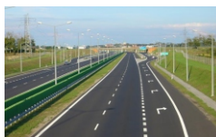
6 National Highways Projects
